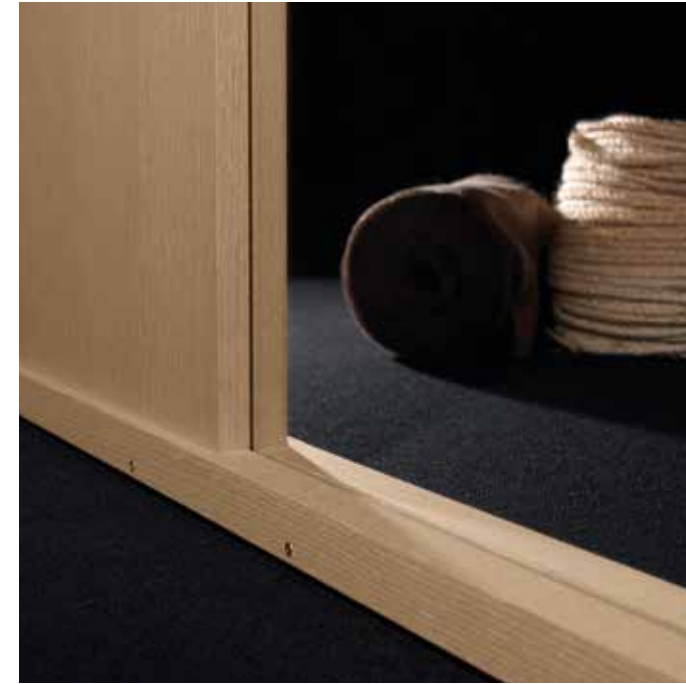
Connessione vetro-legno/ Glass-wood junction
